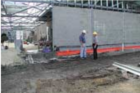
Photo 1 Kordon TB -commercial building
