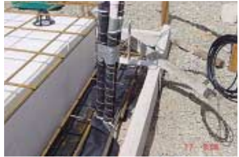
photo 2 showing multiple pipes each protected with Kordon
