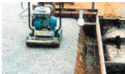
“GranitGard” - being installed under a slab.
