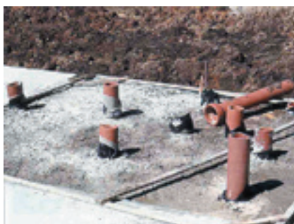
Concrete slab - special attention is required around the service penetrations and joints.
