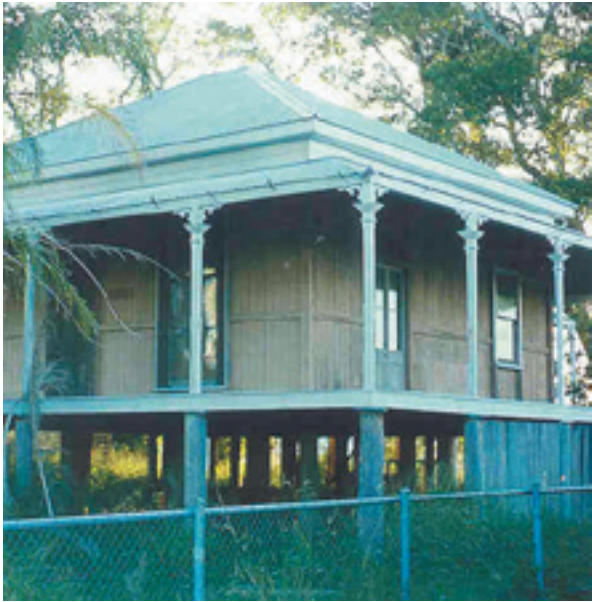
Traditional construction: For over 200 years ground separation has provided effective termite protection.
